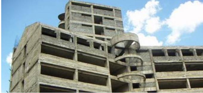
Blue Shield Towers while decommissioned
