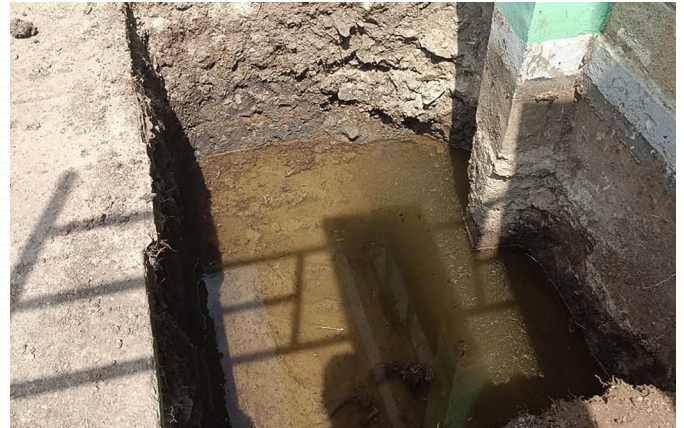
Mater Hospital - Trial Pit
