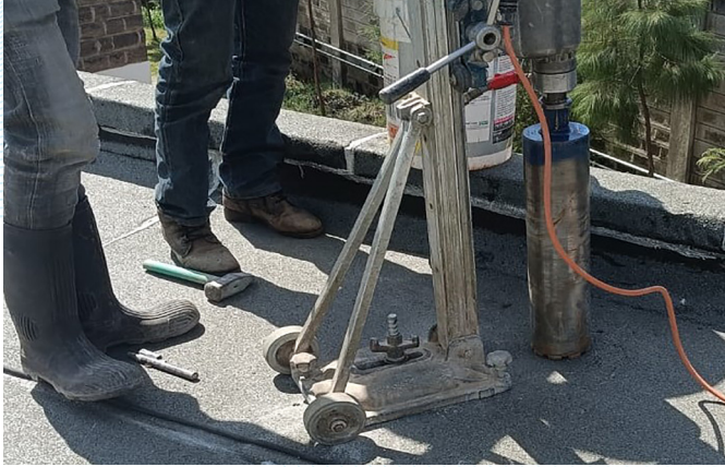
Mater Hospital - Coring
